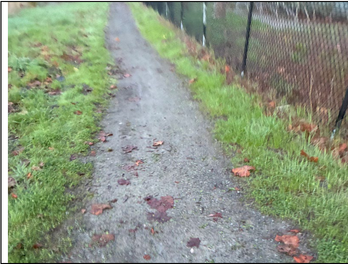
Colgan Creek path between Burgess Drive & Bellevue Ave – consider paving?
