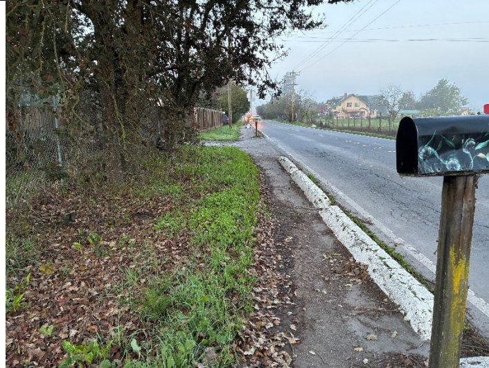
Condition and narrow width of pedestrian pathway/concrete berm on south side of Bellevue Avenue between the Colgan Creek Path and Stony Point Road
