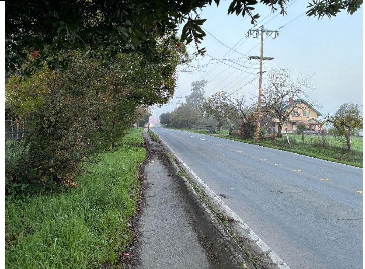
Condition and narrow width of pedestrian pathway/concrete berm on south side of Bellevue Avenue between the Colgan Creek Path and Stony Point Road
